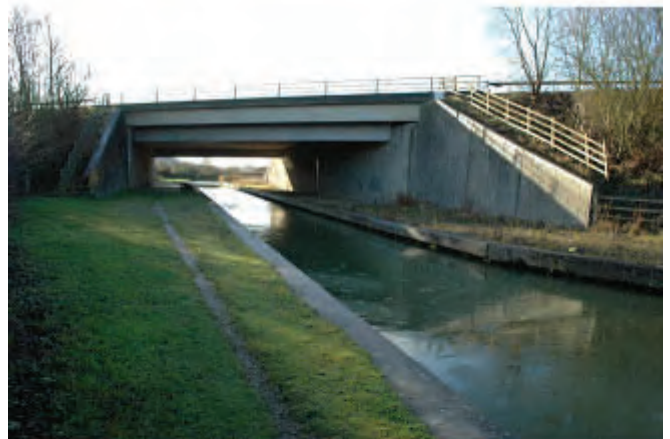
M40 bridge north of Banbury [46]
