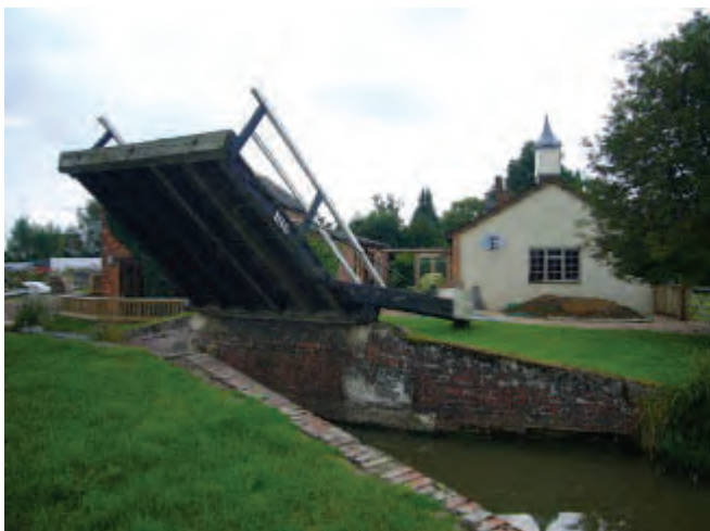
Lift bridge 186 close to Nell's Bridge Lock
