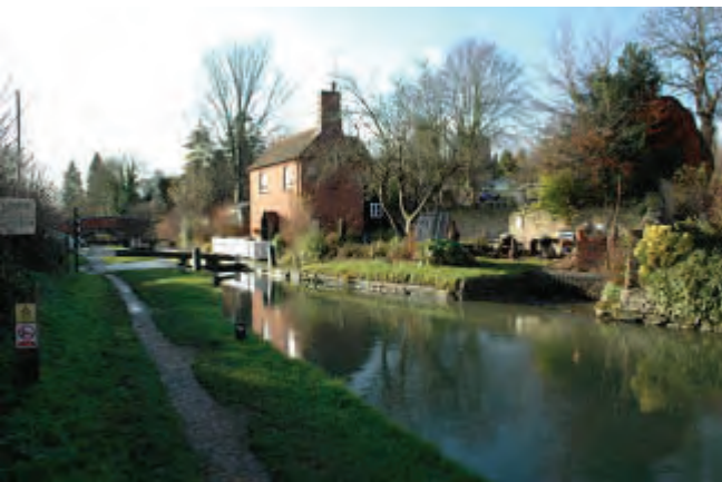
Cropredy Wharf with bridge and outbuildings visible in the distance
