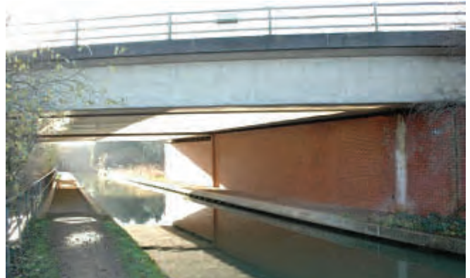
New canal section beneath the Banbury Bypass: distinctly more modern in its appearance, with kerbing and railing to the towpath
