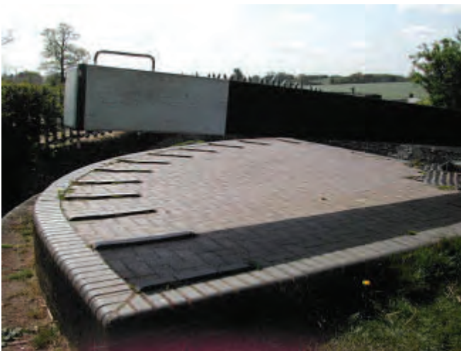
The balance beam at Kings Sutton
