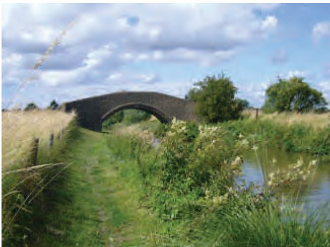
Canal infrastructure sits in the rural landscape near Cropredy
