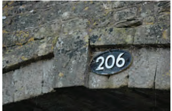
Earlier numbering scheme evident in the key stone of bridge 206
