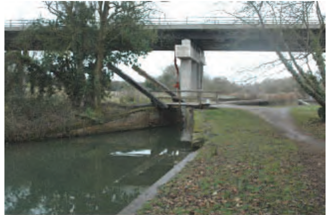
Bridge 233, the Oxford Bypass and southern end of the conservation area
