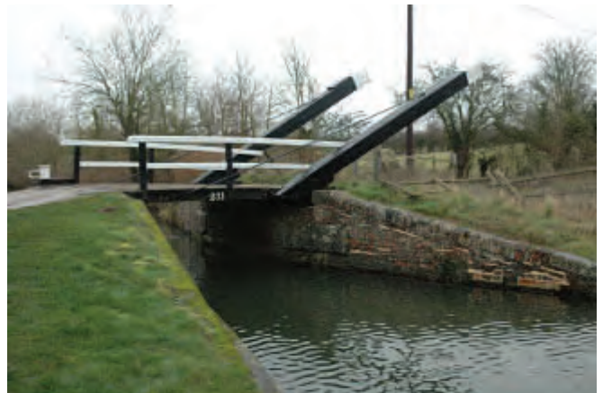
Drinkwaters's Bridge 231: a replacement of the original
