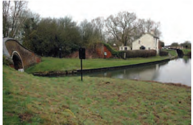
Junction with Duke’s Cut
