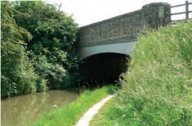
Langford Lane (Bridge 224)
