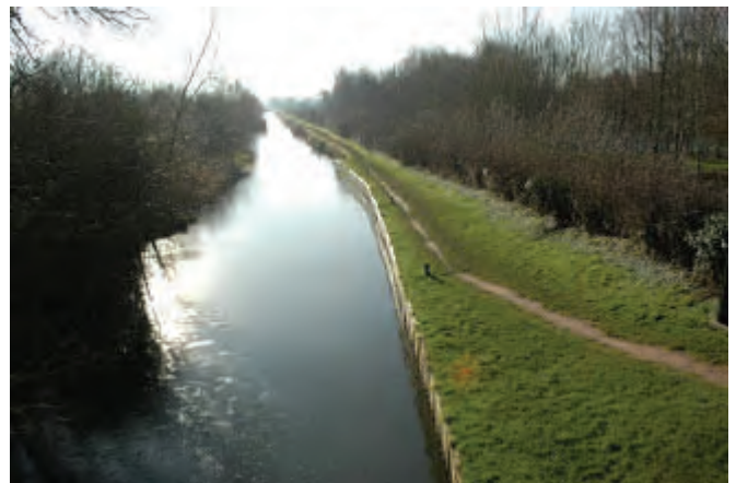
Typical section of canal south from Nell Bridge: the towpath on the right is built up on a low embankment and the hedgerow is quite impervious
