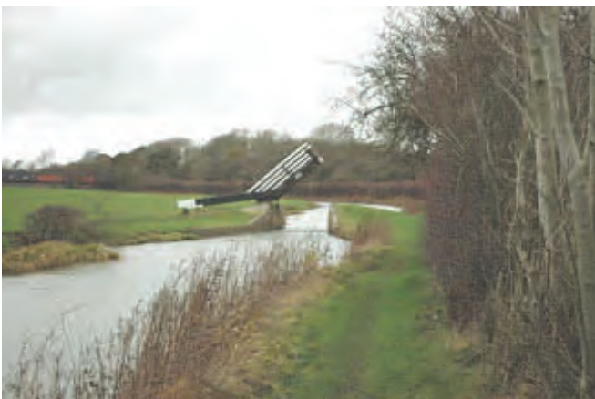
Positive landmark: Boundary Bridge in Warwickshire
