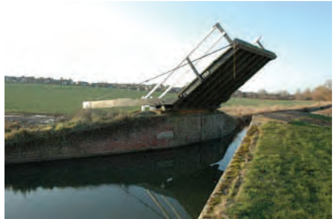
Lift bridge 170, Banbury
