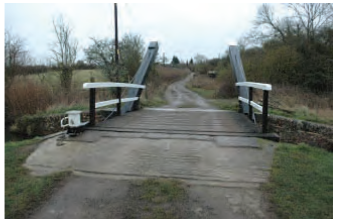
View from Bridge 231
