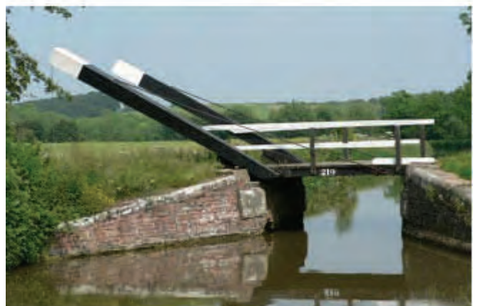
Shipton lift bridge in the closed position
