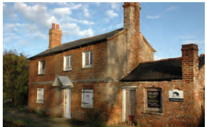
The lock keepers cottage at Little Bourton, little altered since being extended (single storey to the right)
