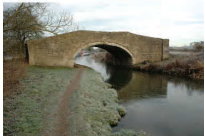
Better quality stonework: relatively unaltered of bridge 207 near Heyford Wharf
