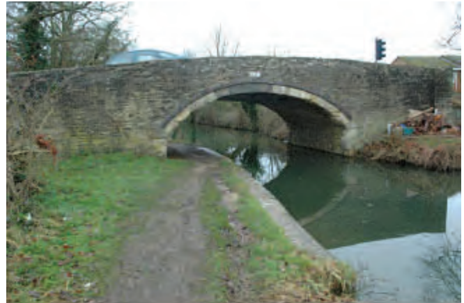
Relatively poor stonework at Yarnton (Bridge 228)
