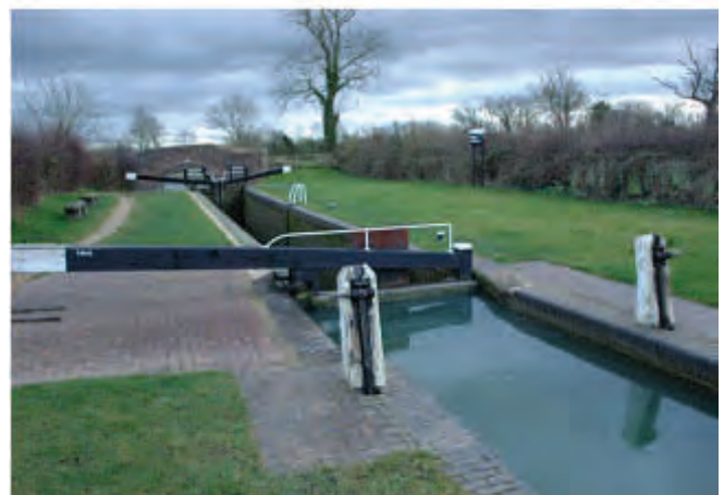
Claydon Middle Lock, typical of those north of Banbury, with double gates at the tail
