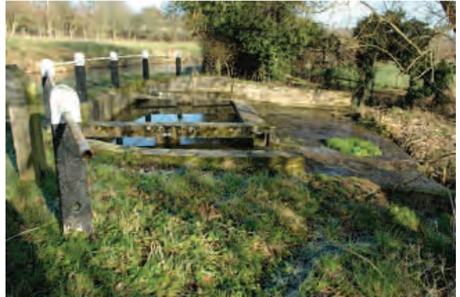
Weir rebuilt in 1940 [86]
