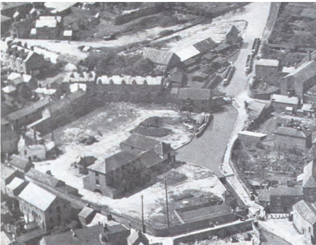
Banbury 1920 showing the Oxford Canal Company warehouse and wharf now filled. Lift bridge 165 is in the foreground with lift bridge 164 with Tooleys boat yard and Castle Wharf behind
