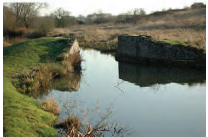
Abutments of former bridge 169
