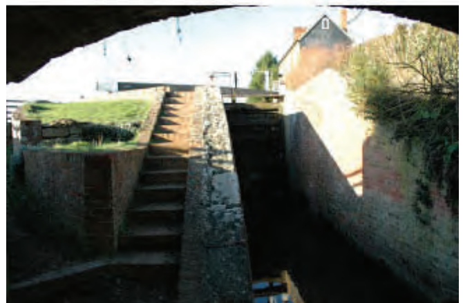
The tail of Somerton Deep showing the single lock gates of locks south of Banbury
