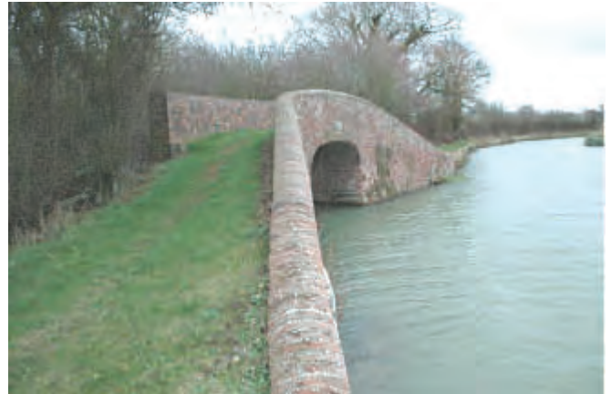
Positive landmark: Tow path bridge over leat
